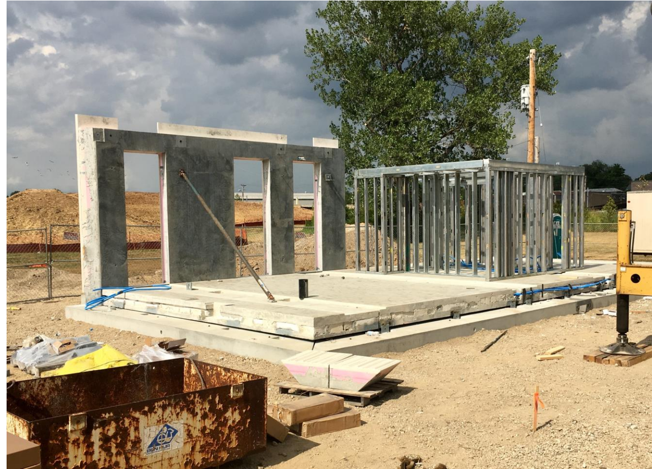
CRETE House Washington University in St. Louis, MO – 2017 US DOE Solar Decathlon Precast Concrete: footings, floors, walls, roof, gutters, planters
