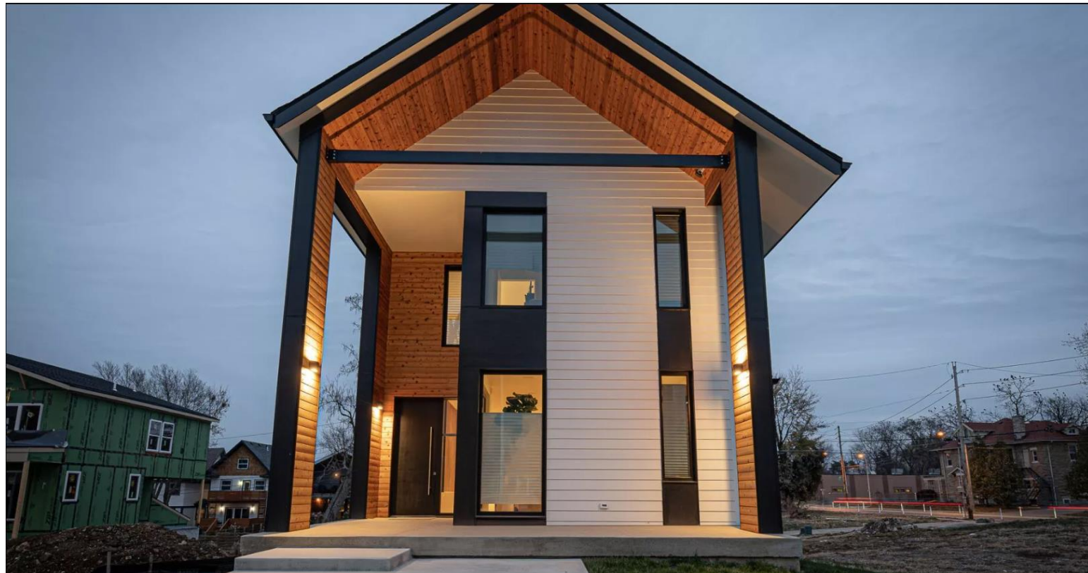
Kala Forest Ave Passive House Kansas City, MO – Phius Core 2021 Certified SIPS w/ Interior Stud Wall, Vented attic Builder: Kala Performance Homes
