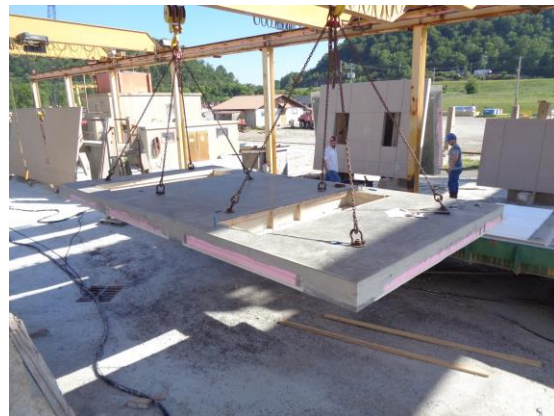
CRETE House Washington University in St. Louis, MO – 2017 US DOE Solar Decathlon Precast Concrete: footings, floors, walls, roof, gutters, planters
