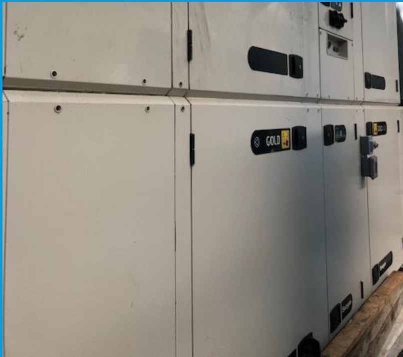
High Efficiency ERV's
